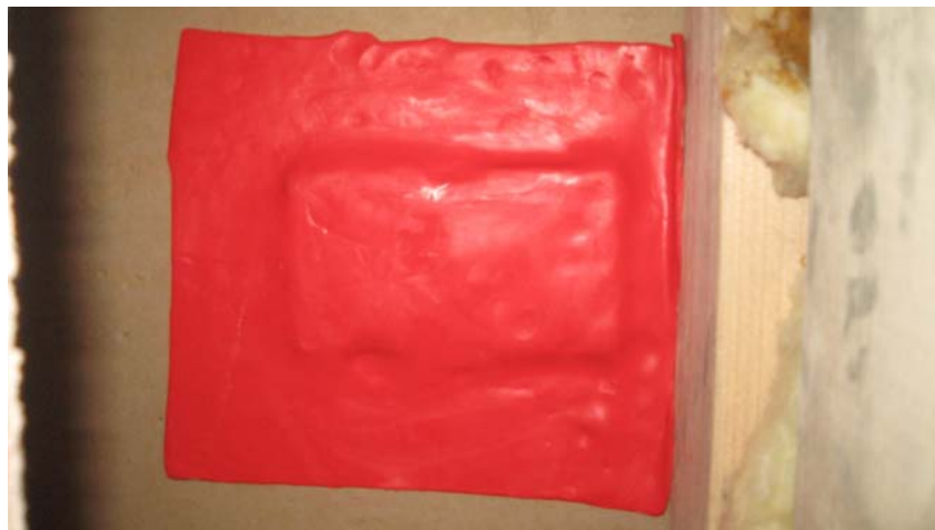
Figure 5 Putty Pad installed outside switch box
