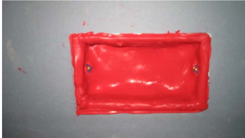
Figure 4 Putty Pad installed inside switch box
