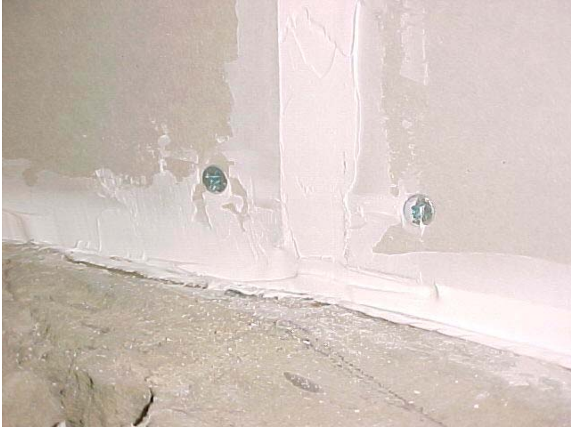
Photograph 4: Fully Sealed Partition Close-Up
